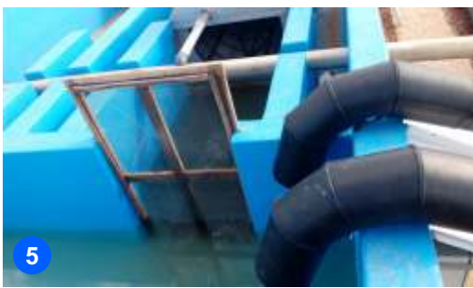
1 400 KLD Aquaculture Wastewater Treatment Plant. 2 Electrochemical Reactors 3 Control Panel 4 Aquaculture Water intake 5 Water Outlet After Treatment
